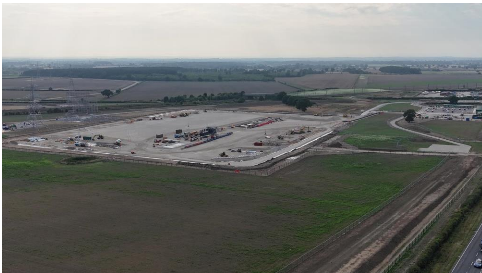
The site for the new Overton electricity substation
